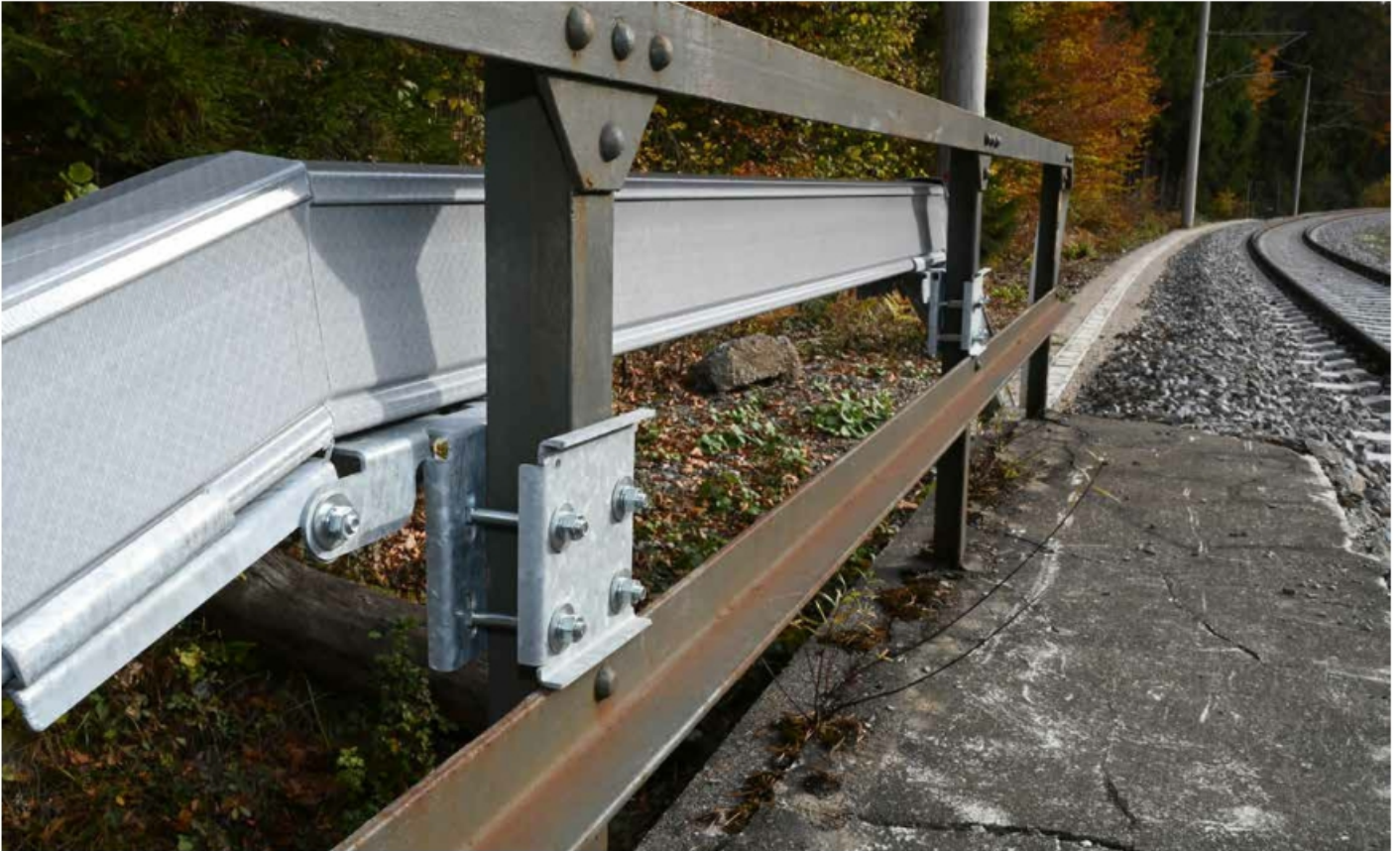
Outhanger standard, hole distance 70-115 mm
