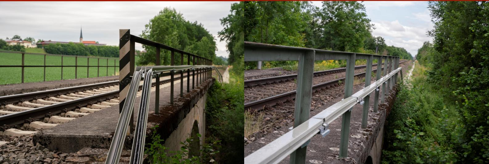
The lightweight and versatile ARCOSYSTEM® is the rail industry's benchmark elevated cable management system, renowned for safely housing power, signal and high-voltage cables. Now, the newly developed SizeZERO® troughing — again manufactured from pultruded fibre-reinforced polymers (FRP) — is designed to fit and protect fibre-optic data cables within a secure, shallower cell of 53mm x 56mm (2952mm<sup>2</sup>).
